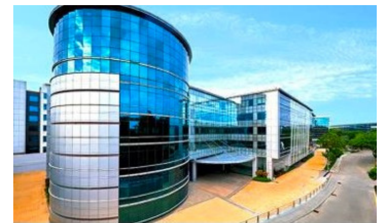
Sunriver, EGL Bengaluru (3,0 lacs sq.ft MEP Refurbishment)
